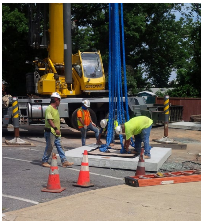
Construction at St. Ambrose Church
