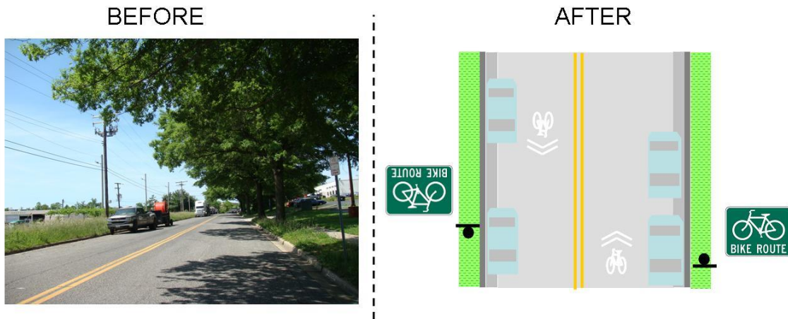
Figure 39: Before and After Signage/Striping Improvements for Staggers Lane
