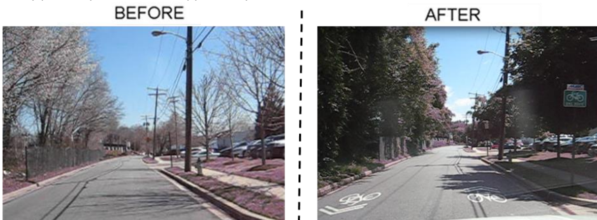
Figure 32: Before and After Signage/Striping Improvements for Lafayette Ave.
